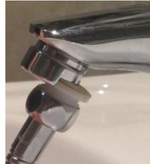
3. Attach the white shower hose connector by screwing onto one end of your shower hose and then push onto the fitted tap aerator. On first use, only turn the water on slightly to ensure the seal is watertight.
